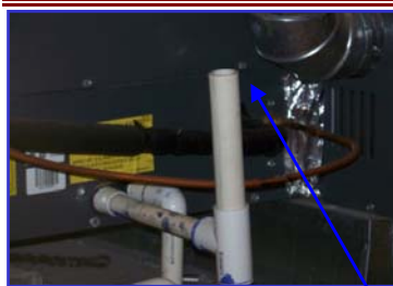
Missing cap over PVC drain pipes
